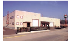
NEW WAREHOUSES RUBÍ, BARCELONA
